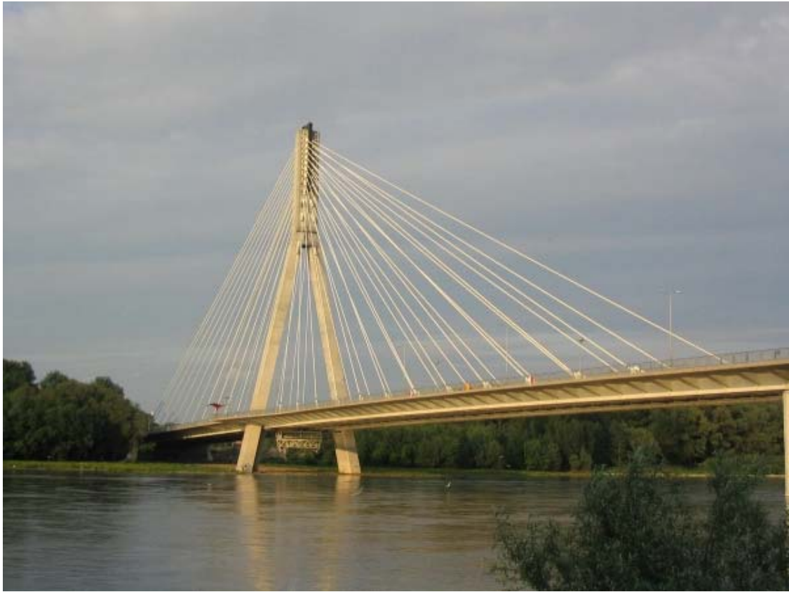
Fig. 3. Swietokrzyski Bridge over Vistula River in Warsaw
