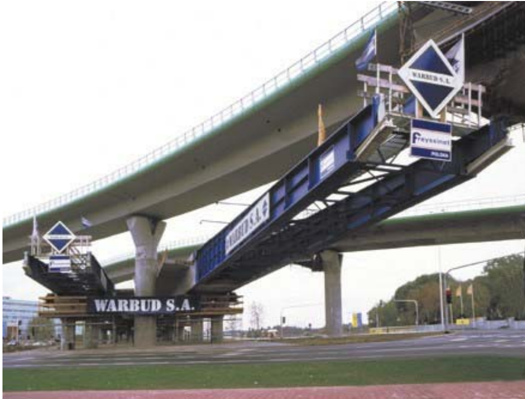
Fig. 11. Czerniakowska interchange Bridge in Warsaw
