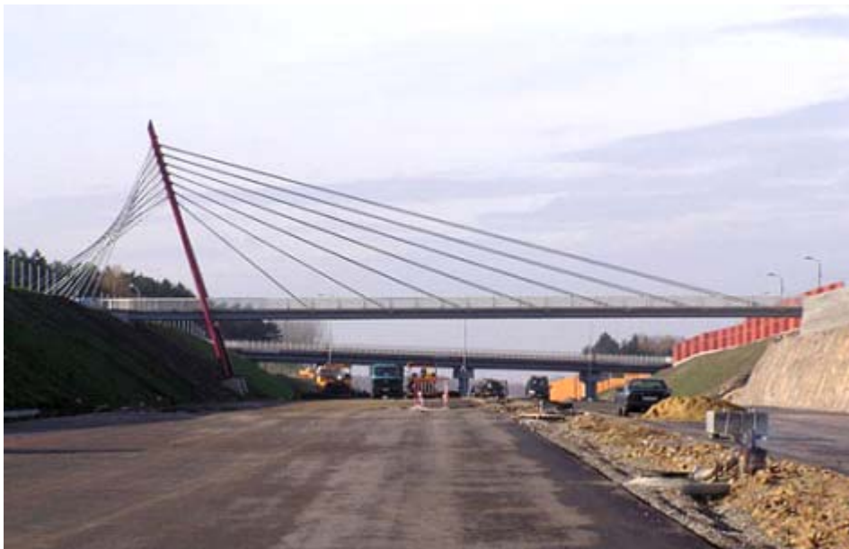
Fig. 13. Footbridge over A4 motorway in Ruda Śląska
