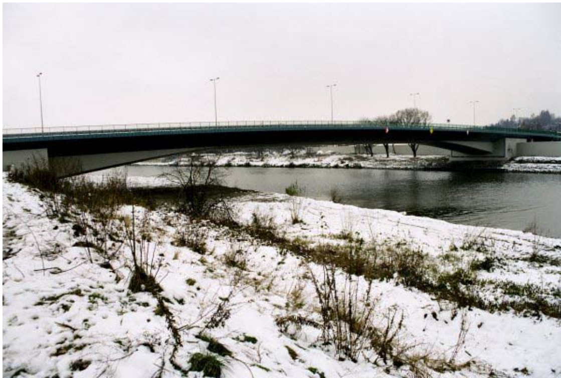
Fig. 10. Zwierzyniecki Bridge over Vistula River in Cracow [18]
