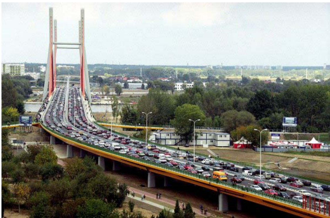
Fig. 4. Siekierkowski Bridge over Vistula River in Warsaw
