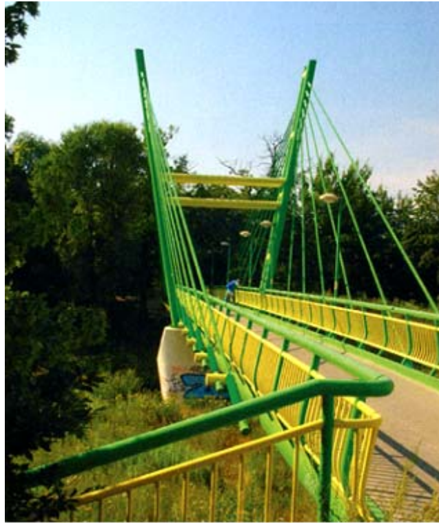
Fig. 12. Lesnica Footbridge in Wrocław
