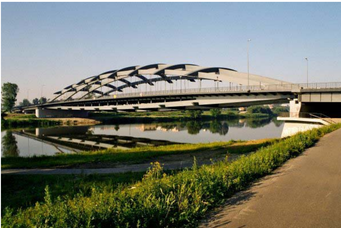
Fig. 8. Kotlarski Bridge over Vistula River in Cracow [18]
