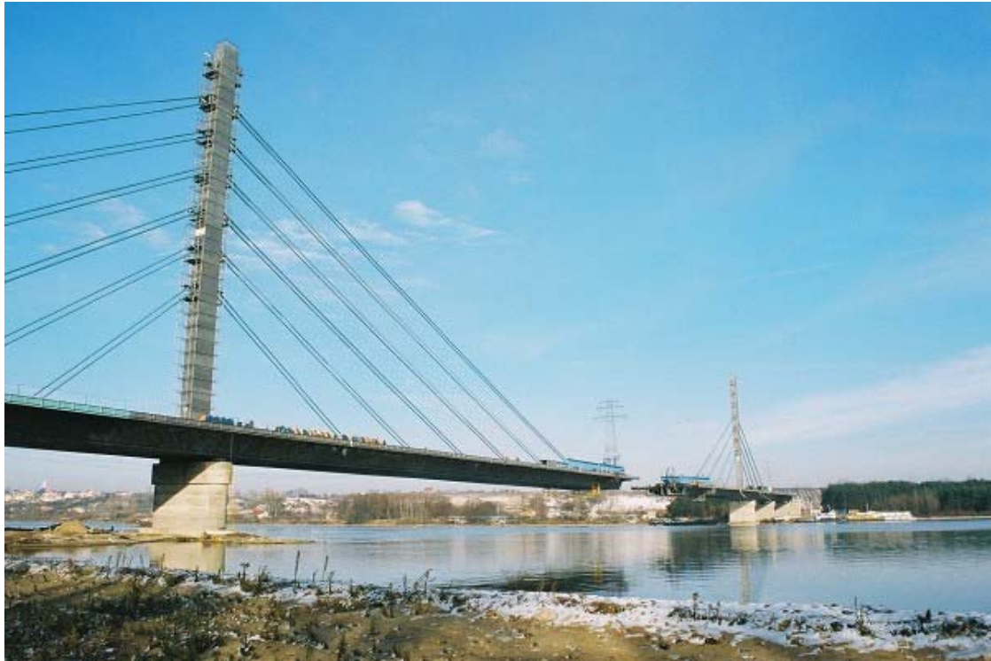
Fig. 7. New Plock Bridge over Vistula River in Plock
